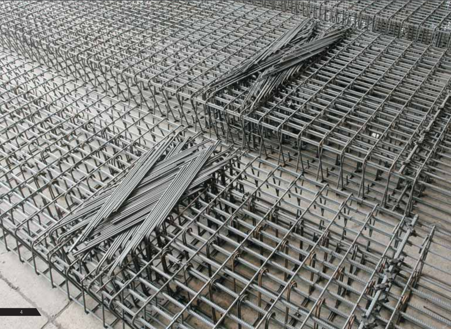
Prefabricated diaphragm wall cages
