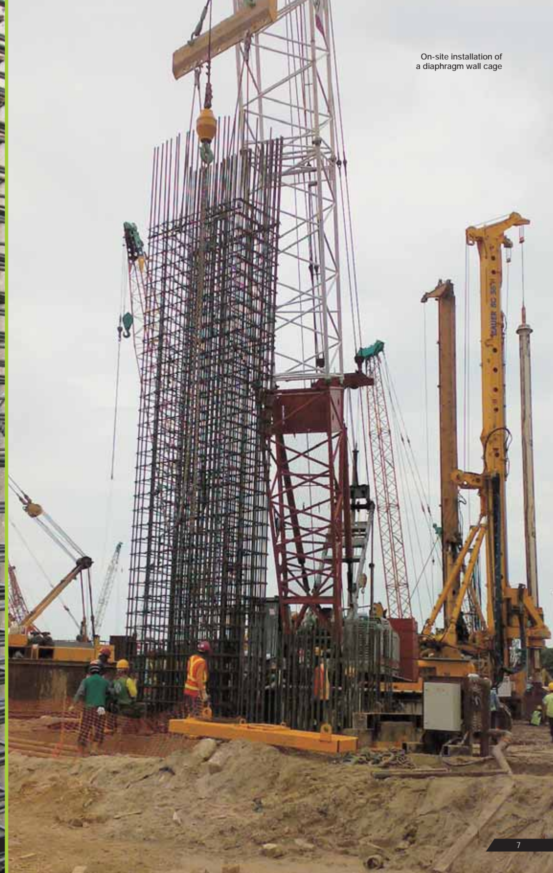
Diaphragm wall cage
