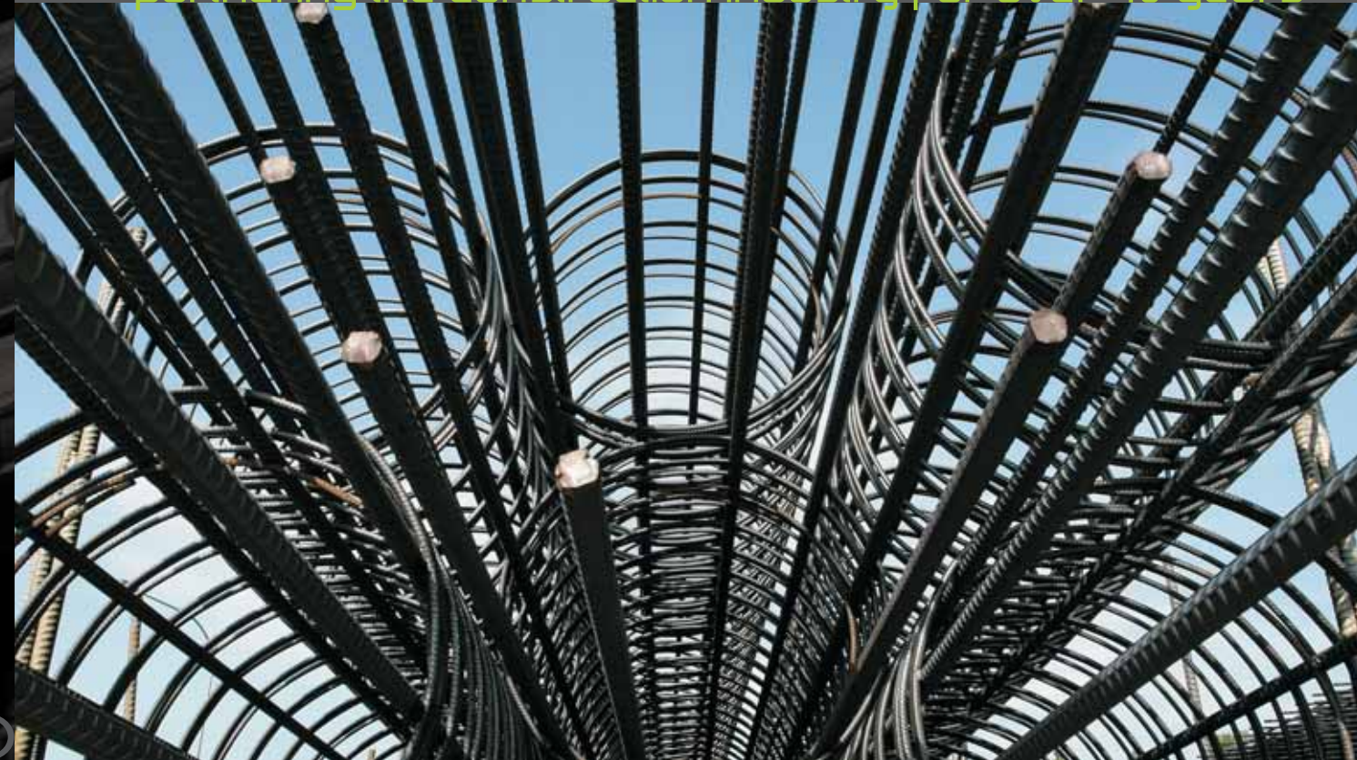
Bored pile cages are used for foundation works.
